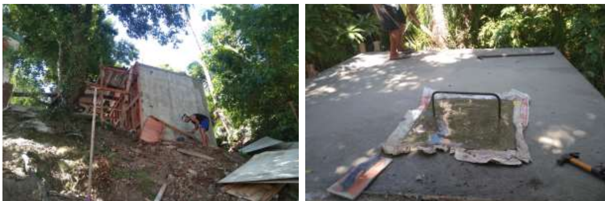
Concreted ground reservoir in Brgy. Catadman
